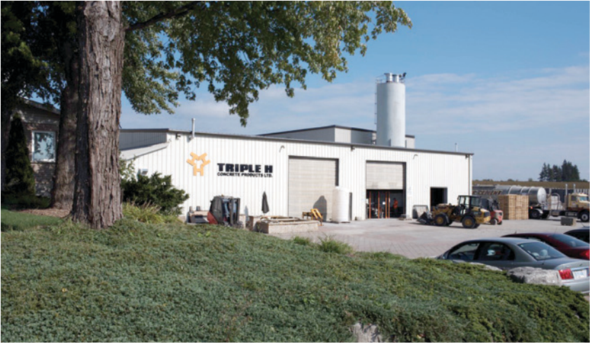
Home of Triple H Concrete Products
