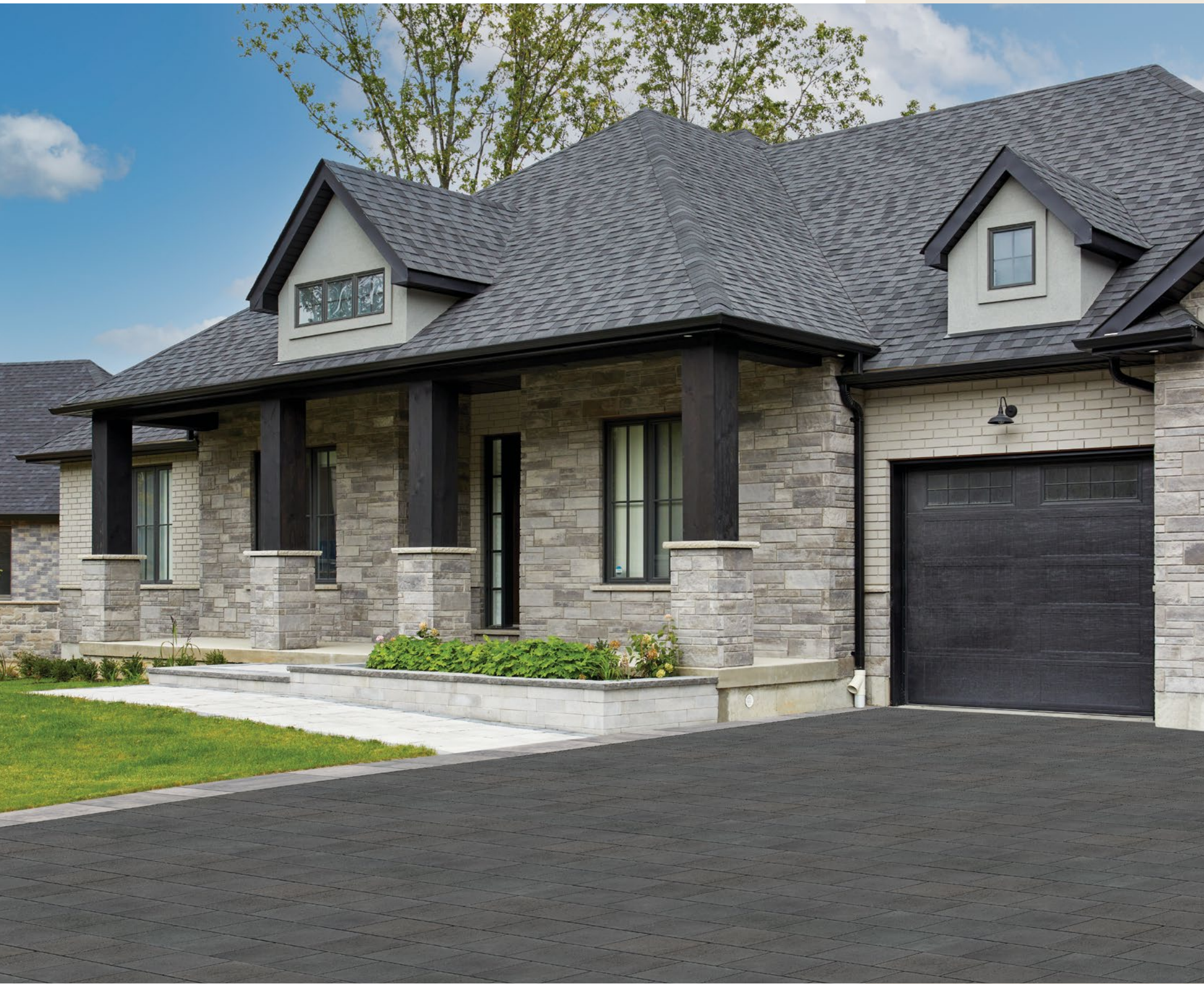
Stone Masonry: Granada, Ashland with Contempo, Dover (PRP) Pavers: Nueva® Paver, Onyx with Rialto 80mm, Marble Grey border
